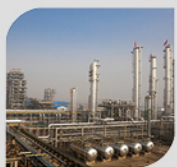
Energy and chemical equipment
